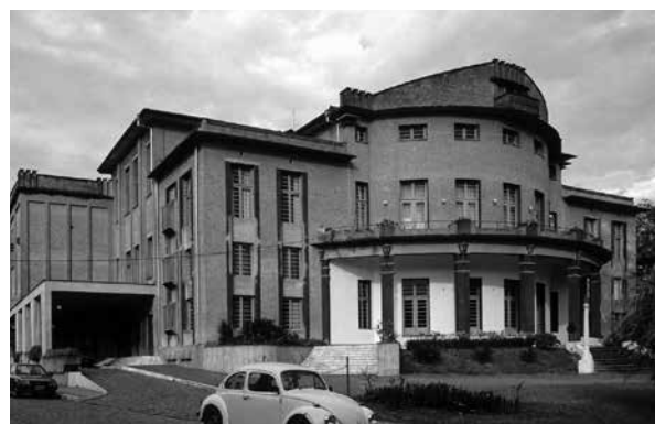
Fig.10 Carlos Gomes Theater, city of Blumenau, state of Santa Catarina, Brazil.
