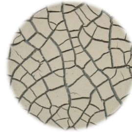
Fig. 1 Desiccation cracking pattern of soil.
