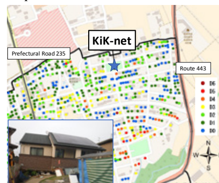
Figure 3. Collapsed building near the KiK-net station.
