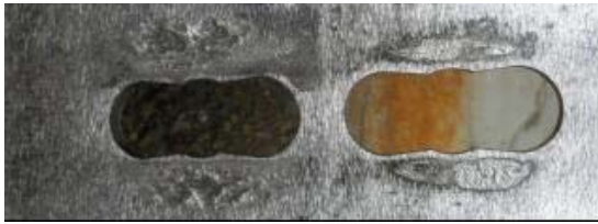
Figure 13 Abrasive marks on the contact surface of splice plate near slotted bolt holes caused by 480 cycle's frictions.
