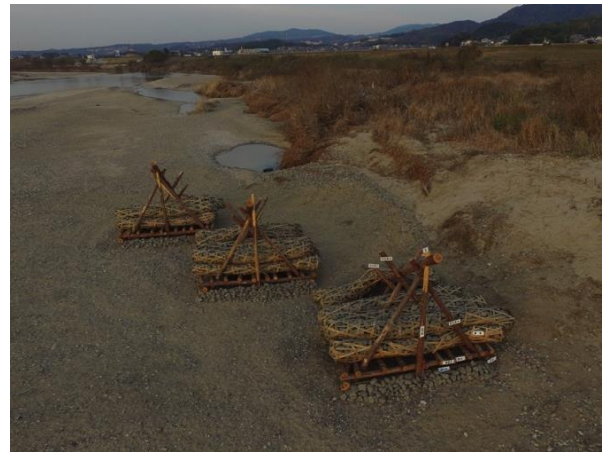
Photo 1 “Seigyū” (crib spur) set up in the Kizu River as a test trial in December 2017
