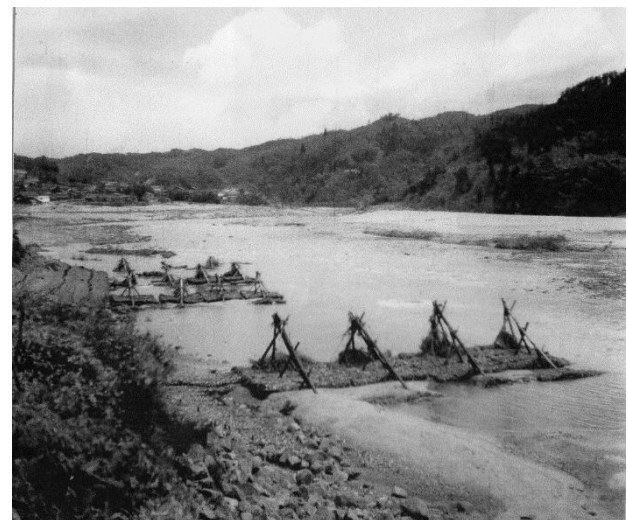
Photo 2 Seigyū (crib spur) in the Kizu River in 1953 (Photo taken by Horii. Courtesy of Nakatsugawa and Fukui)
