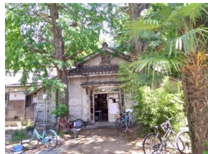
pic. 1 - Entrance to Yoshida Dormitory
