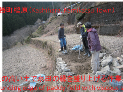
Figure 25: Piling stones and mounding edge of paddy fields with viscous soil
