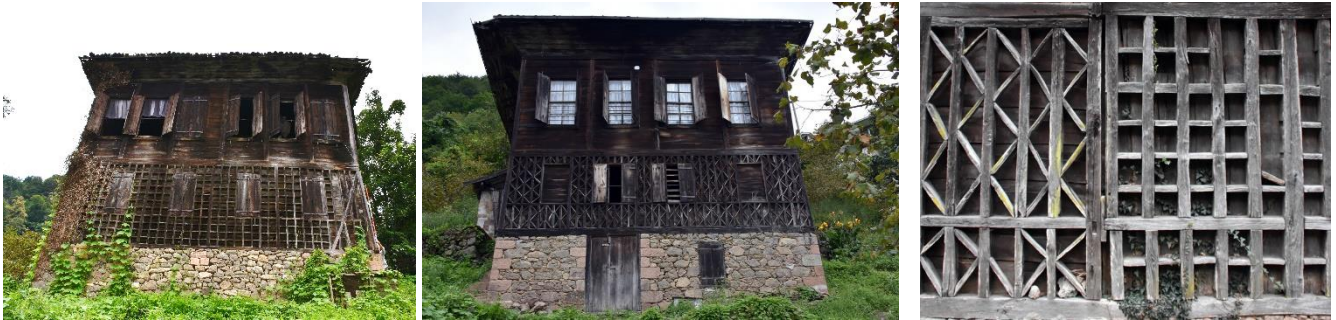
Figure 3.17 Mixed construction system in Karacakaya and Üstündal (Var, 2017).
