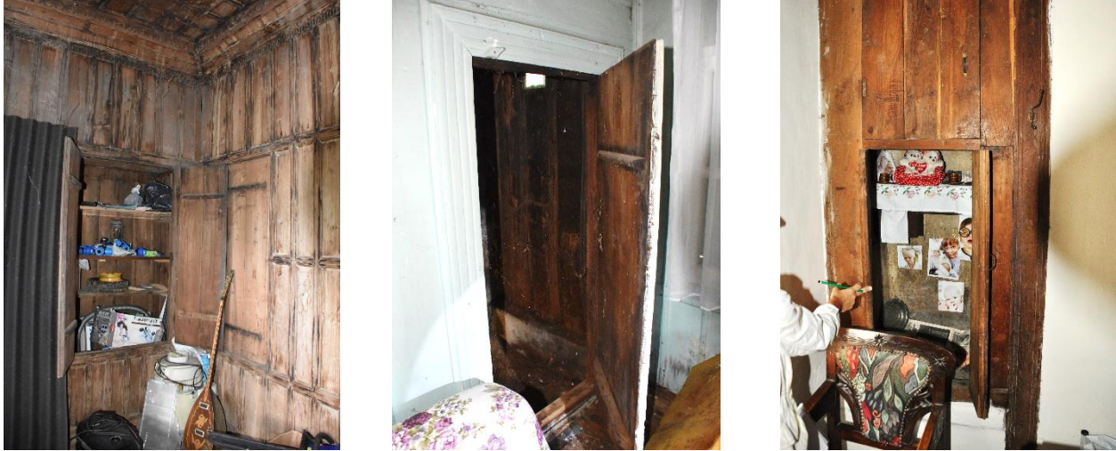
Figure 3.20 Built-in cupboards in the existing vernacular houses in Karacakaya, and Üstündal (Var, 2016).
