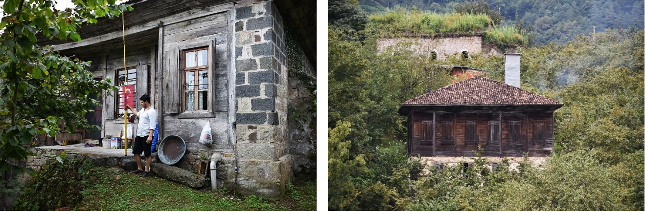
Figure 3.14 Timber masonry ( yontma ahşap yığma ) houses in Karacakaya (left) and in Üstündal (right), (Var, 2017).
