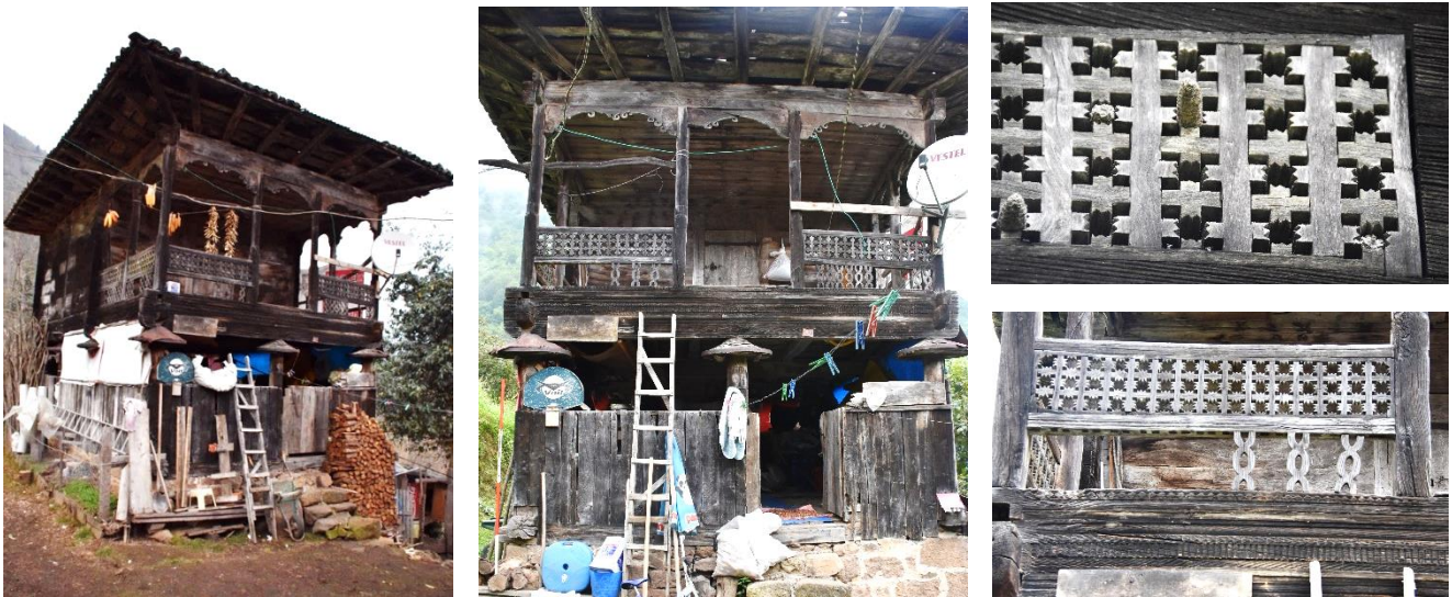
Figure 3.21 Details of a serander in Karacakaya Village, Sürmene (Var, 2016).
