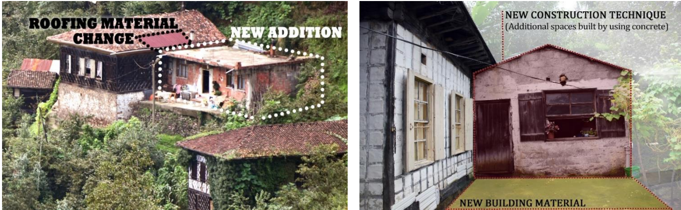
Figure 4.14 Additions to a vernacular house in Üstündal Village (2016).
