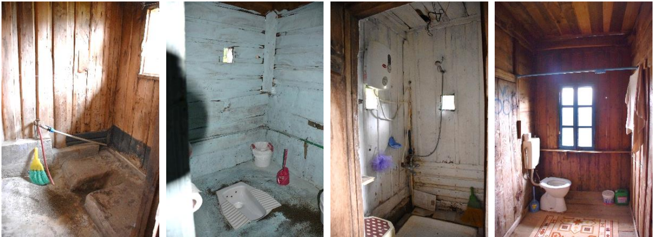
Figure 4.9 Different examples of toilet and bathroom facilities. (1): Original toilet, (2): Traditional toilet – new fixture, (3): New bathroom, (4): New toilet fixture.
