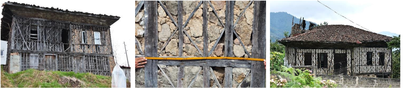
Figure 3.16 Vernacular house with muskalı system & details; vernacular house with çatakura system (Var, 2017).
