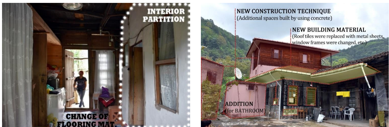
Figure 4.7 Spatial changes in a vernacular house in Üstündal: interior (left) and exterior (right).
