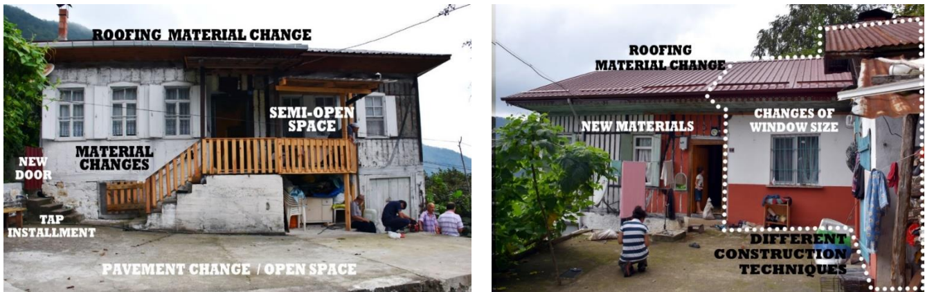
Figure 4.13 Morphological changes in a vernacular house in Karacakaya (left) and in Üstündal (right; 2016).
