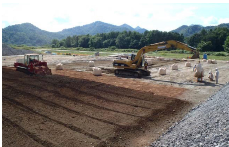
Fig. 1.2 Construction site of sorption layer method (Technical Committee of Environmental Conservation Technology Association, Hokkaido 2012)
