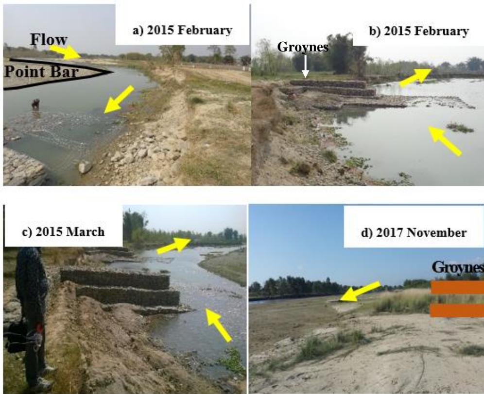
Photo 1.3 Bank erosion and implementation of groynes in the channel shown in photo 1.2
