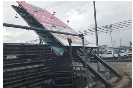
Fig.44 damage to a water-based solar system (科研費報告書, 2019)
