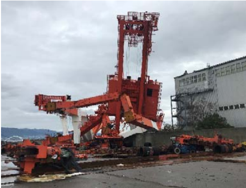
Fig.49 gantry crane collapse (科研費報告書, 2019)
