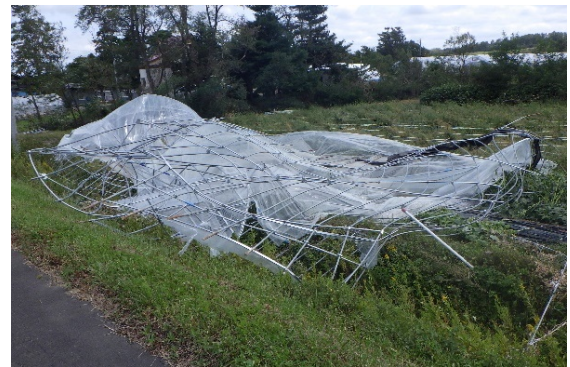
Fig.45 collapse of a pipe house (科研費報告書, 2019)
