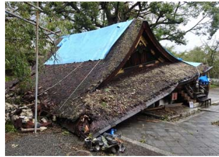
Fig.38 collapse of a Shinto shrine (科研費報告書, 2019)
