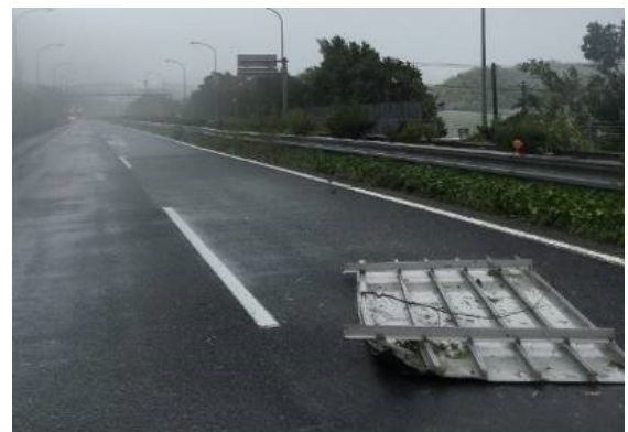
Fig.47 sign-board blown out by wind (科研費報告書, 2019)
