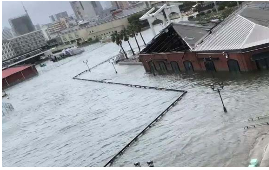
Fig.58 Inundation at Harbor Land in Kobe ((Twitter 9/4 14:26)
