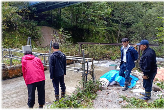
Photo 7 Sediment measurement facilities in Hodaka Laboratory.
