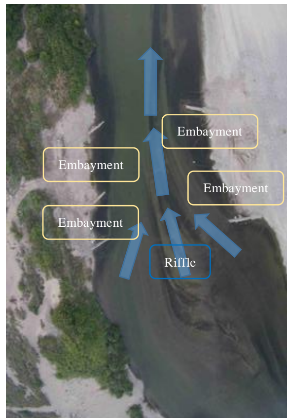
Fig. 2 River bed topography after installation of groins using bamboogabions
