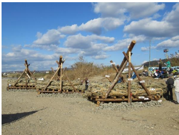
Photo 6 Seigyu (crib spur) set up in the Kizu River
