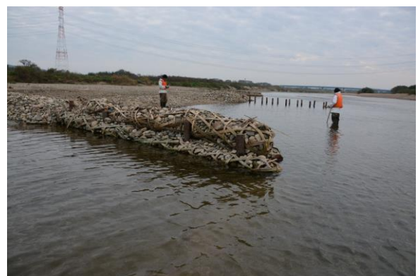
Photo 4 Groins using bamboo gabion in the Kizu River (2015/11/22)
