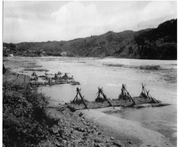
Photo 7 Seigyū in the Kizu River in 1950s (Photo taken by Horii. Courtesy of Nakatsugawa and Fukui)
