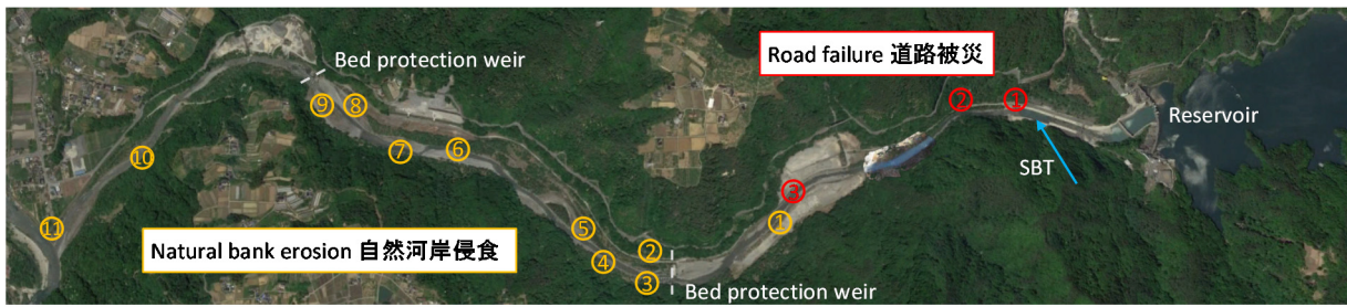
Fig. 4 Location of bank erosion in the downstream of Koshibu Dam in July 2018.
