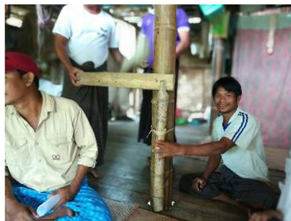
Fig. 6. Floor adjustment in a bamboo house.
