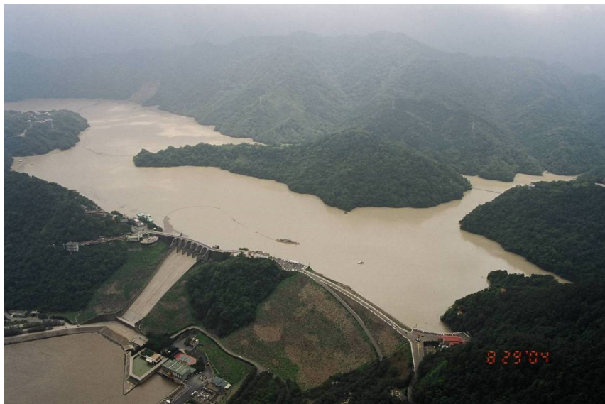
Figure 6: Typhoon Aere caused muddy in Shihmen Reservoir in 2004
