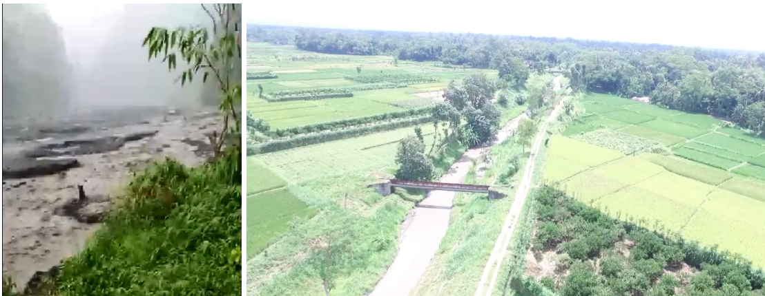
Fig. 7: Sediment laden flood in upstream of Putih River in November 2016 (left) and condition of existing Putih River sediment bypass channel in February 2017 (right)
