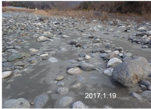
Figure 12: Riverbed at junction with Tenryu River after test operation
