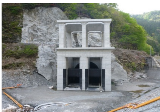
Figure 5: Inlet structure: front (left), with sub-gates above main gates, and in cross-section (right)
