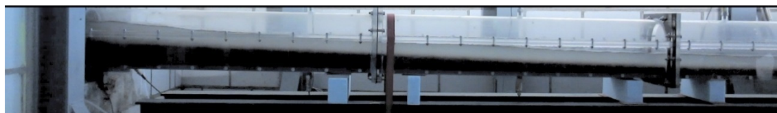
Fig. 14: Side view on the SBT free-surface flow with Q_{SBT} = 150 \text{ m}^3/\text{s} during drawdown for the additional flushing after large sediment deposits have been formed in the u/s reservoir. The flushing efficiency in the reservoir and sediment transport in the SBT are high at the beginning of the flushing test. The sediment aggradation in the SBT reaches a constant slope of about 4%. At the end of the test, the SBT is cleared from these deposits. Although the deposits in the SBT are high, free-flow conditions prevail (from VAW 2016).
