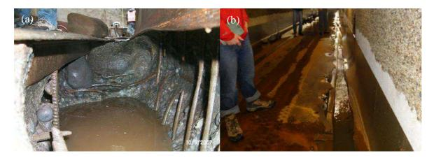
Figure 2: Abrasion patterns in the steel lining of Mud Mountain SBT, a) photograph in 2007: damage expanded into the concrete proof lining below the steel plate, b) photograph in 2015: longitudinal abrasion channel along the side wall (USACE 2016).
