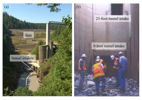
Figure 1: a) Photograph of Mud Mountain dam and tunnel intake structures in 2012 (courtesy of Mike Betz), b) photograph of tunnel intakes with gravel deposition (USACE 2016).
