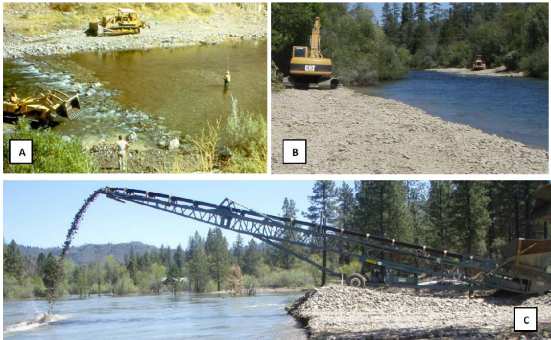
Fig. 2: Coarse sediment augmentation photographs. A) Construction of the first artificial spawning bed in 1972 at a river mile of 112.0 from its river mouth (RM 112.0). Photograph shows low-flow placement of oversize sediment used for grade control structure and coarse sediment augmentation for the artificial riffle; B) Low-flow placement of coarse sediment in the form of constructed point bars in 2009 (RM 110.4); C) High-flow injection of coarse sediment in 2011 (RM 104.9). Photos are from Krause (2012).
