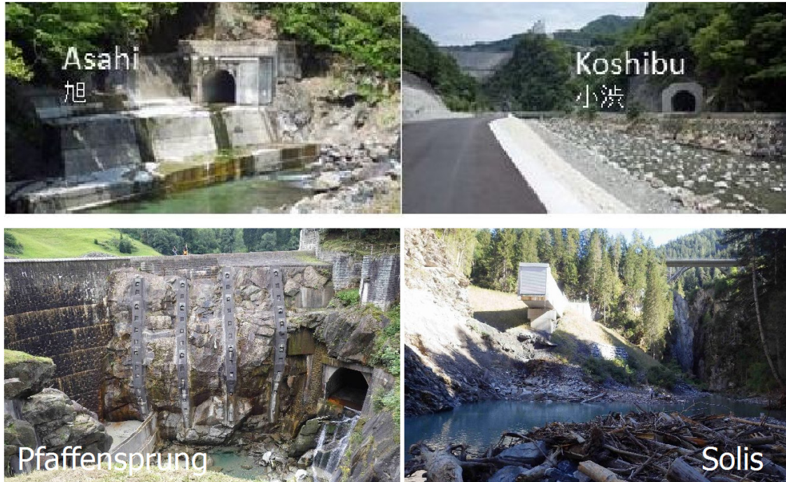
Fig. 1: Asahi and Koshibu in Japan and Pfaffensprung and Solis in Switzerland. Sediment bypass tunnels were installed at Asahi in 1998, Koshibu in 2016, Pfaffensprung in 1922, and Solis in 2012. Photos in Japan are from Awazu et al. (2015).
