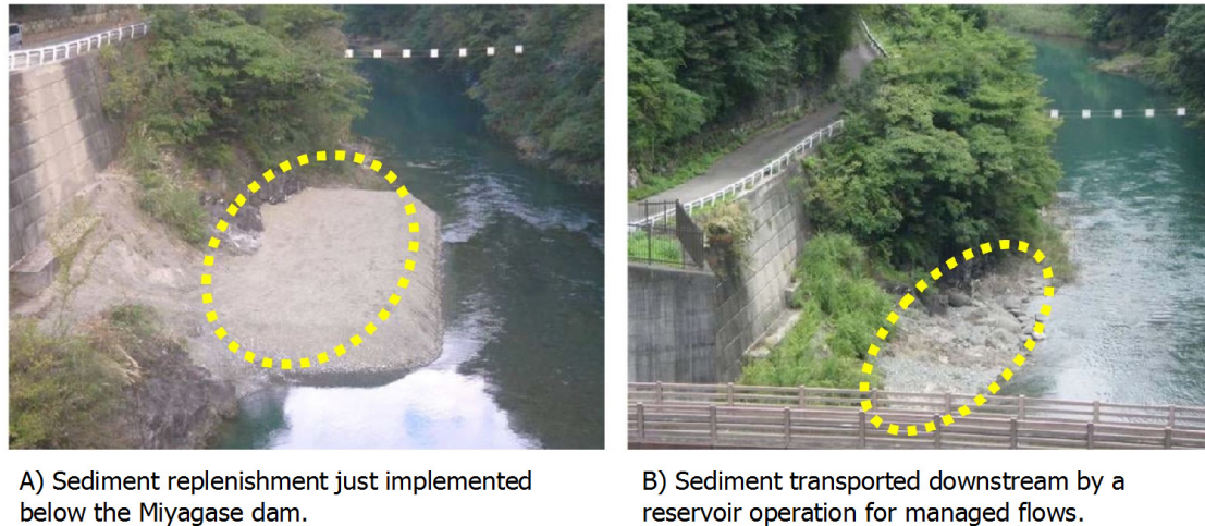
Fig. 3: Sediment replenishment at the Miyagase dam. (SRBC 2015) Approximately 200 m 3 of sediment was replenished on the riverbed at the downstream of Miyagase. The sediment was flushed away after a flood event. At the Miyagase dam, a reservoir operation for managed flows was also implemented with the view to detaching the attached algae.
