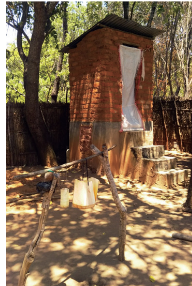
Figure 6. Ecosan toilet constructed by the NICCO Malawi Ecosan project. (Taken by the author)
