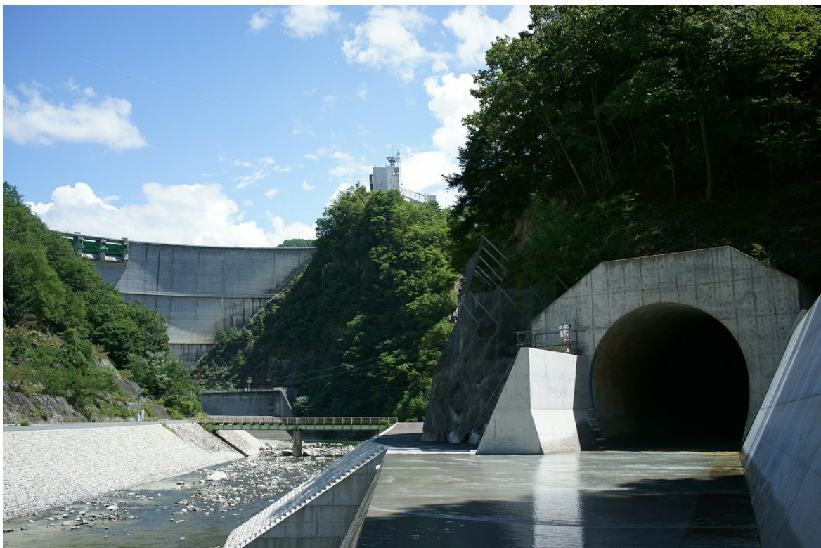
Fig. 2.6 The Koshiybu dam and the SBT outlet.
