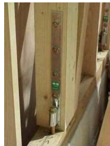
Fig.6 Example of “hold-down connector” set at column-sill joint in a wooden conventional post & beam structure. This connector, for example, can be used to sustain 20kN pullout force.
