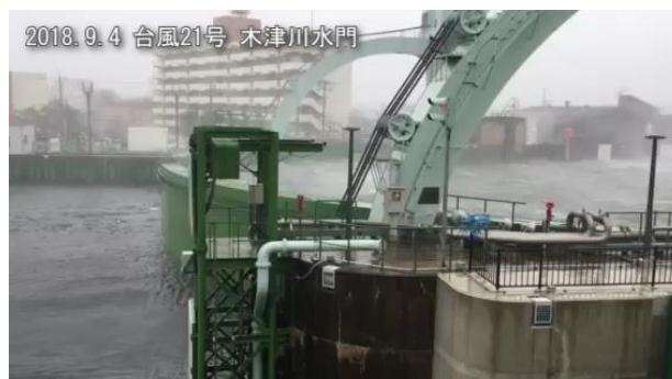
Fig.4 Prevention of Storm Surge on September 4, 2018 ( presented by Osaka Prefecture)
