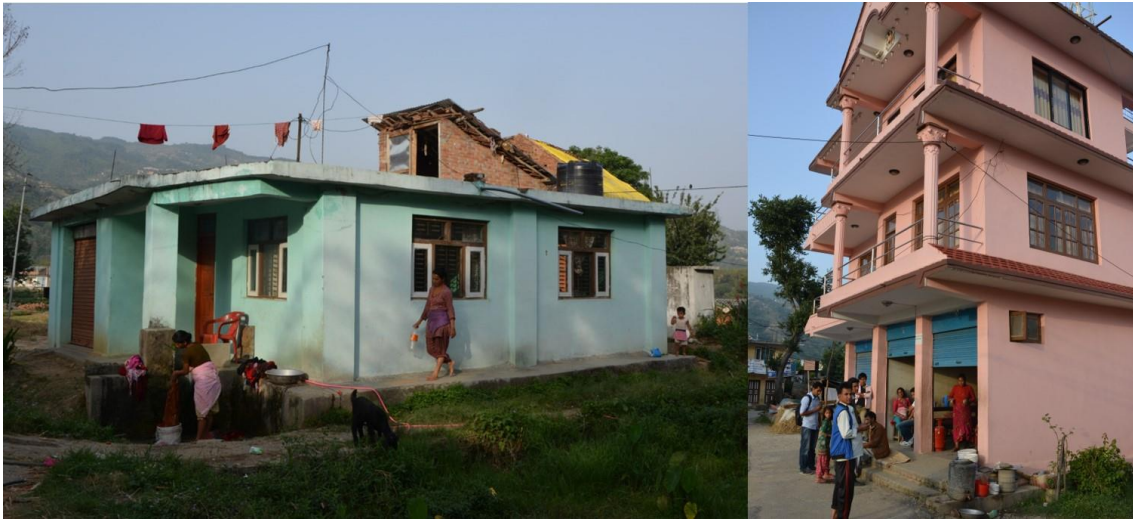
Figure 8. The retrofitted houses in Aalapot sustained no damage (Left: newly constructed house based on the advice, right: Student C's retrofitted house)
