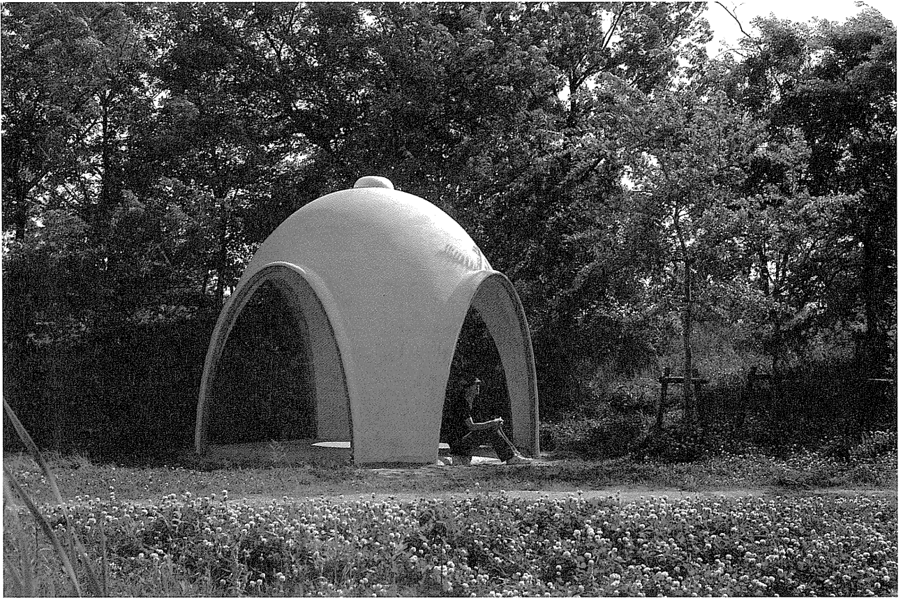
SAKAN Shell Structure Project 実大実験棟, 2006-2007
