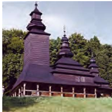
Pic. 7-b Ukrainian Lemko type blockhouse church with upper beam-pillar part of the narthex belfry. Kanora village, 18th c.
