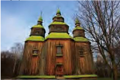
Pic. 4-c Zalom space-construction shape on an octagonal cage base, Zarubintsy village church.
