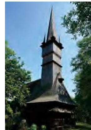
Pic. 7-c Romanian blockhouse church with upper beam-pillar part of the narthex belfry and rafter roof. Ukrainian Krainikove and Romanian Surdesti villages, 17-18th c.
