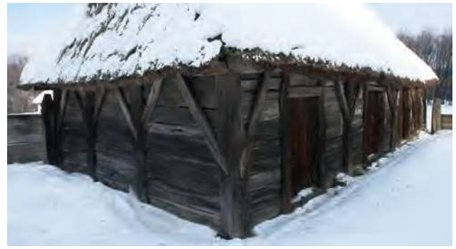
Pic. 8 Hybridized form of beam-pillar and blockhouse system mixing. Rural houses and household outbuildings of Carpathian region (18-19th c.).
