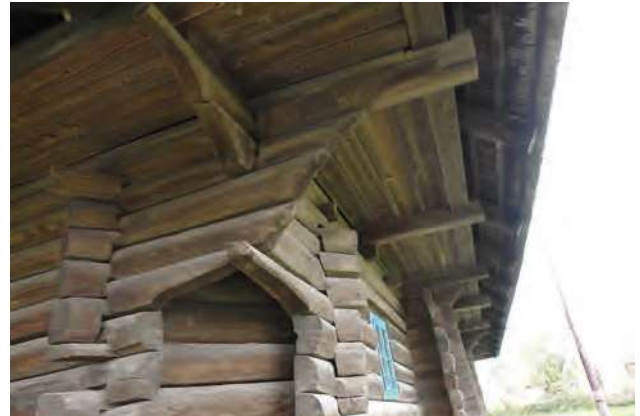
Pic. 8 Hybridized form of beam-pillar and blockhouse system mixing. Rural houses and household outbuildings of Carpathian region (18-19th c.).
