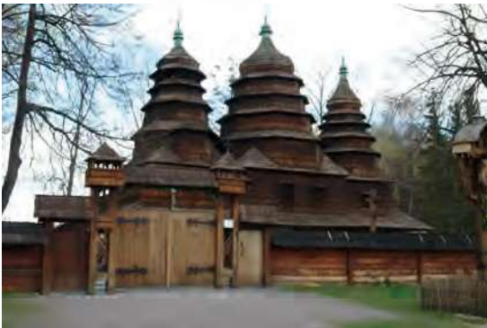
Pic. 7-a Ukrainian Boyko type blockhouse church with upper beam-pillar part of the narthex belfry. Sukhyi and Kryvka villages, 18th c.
