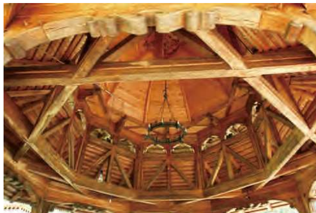
Pic. 9-b Close to the timbers multiplied octagon-on-square structures of beam-pillar framing (Romania, summer altar at Barsana monastery).
