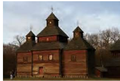
Pic. 4-b Zalom space-construction shape on a square cage base, Kisorychi village church.
