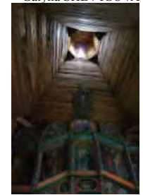
Pic. 4-b Zalom space-construction shape on a square cage base, Kisorychi village church.
