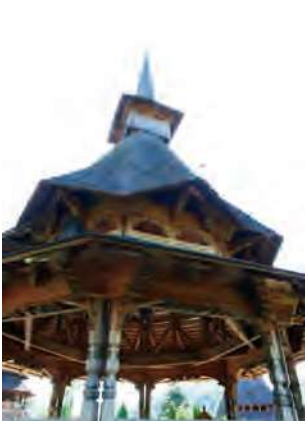
Pic. 9-b Close to the timbers multiplied octagon-on-square structures of beam-pillar framing (Romania, summer altar at Barsana monastery).
