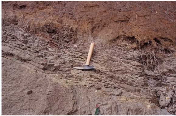
Fig. 3 Exfoliation of vapor-phase crystallized ignimbrite due to weathering (Chigira et al., 2002).
