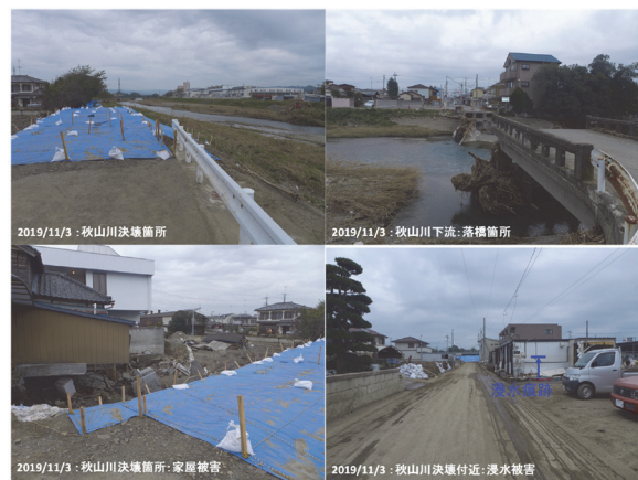
Fig. 5 Levee breaching points along the Akiyama River (photos are taken by the author on Nov. 3, 2019)
