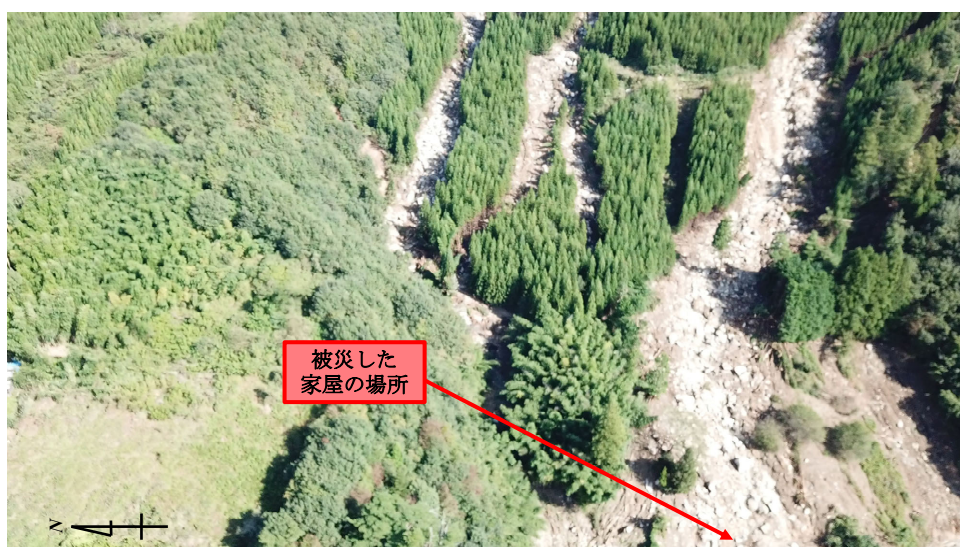
Fig. 5 Erosion by debris flow at the upstream of the damaged house
