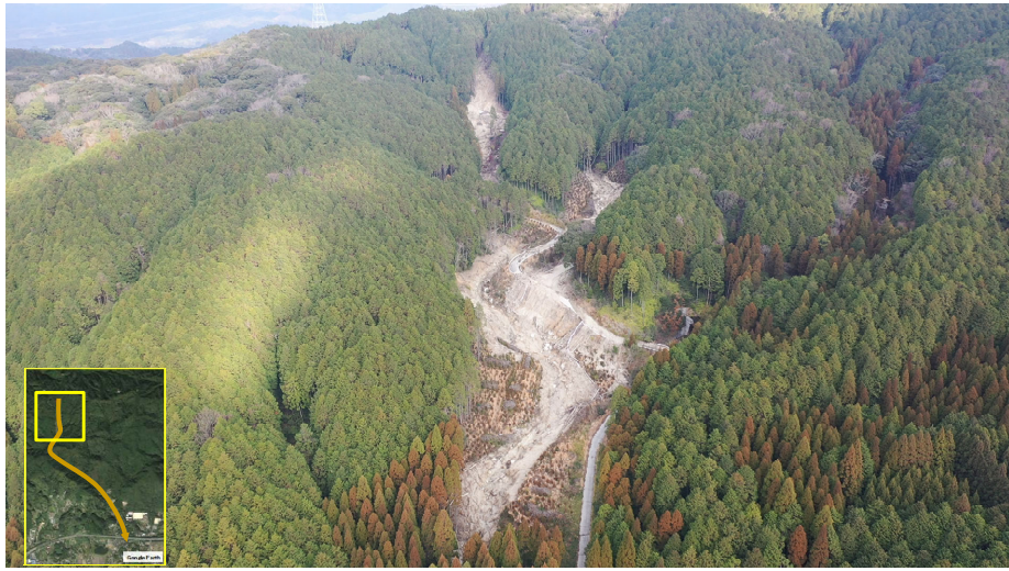
Fig. 12 Confluence of valleys and wide channel width area
