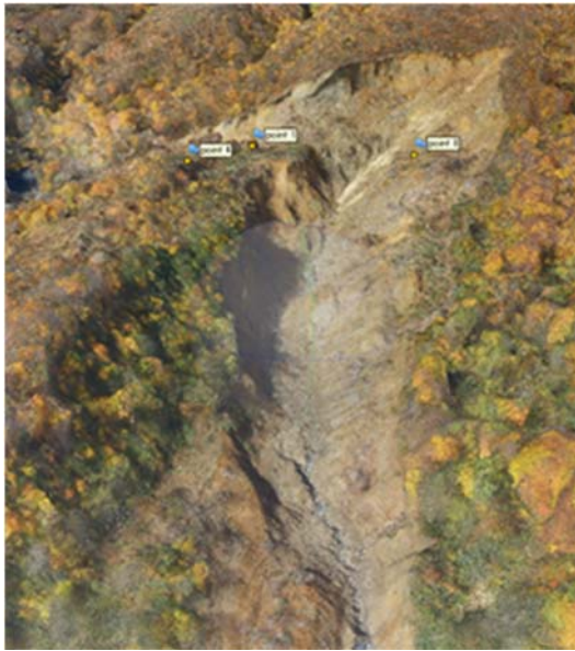
Fig. 1 Orthomosaic image in a Landslide in Iiyama, Nagano.
