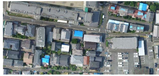
Fig. 4 Roofs covered by blue-sheet Ibaraki City, Osaka.
