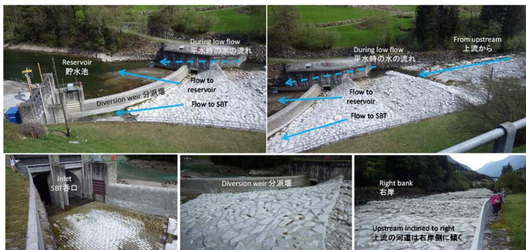
Fig. 11 Diversion weir and SBT inlet of Pfaffensprung Dam in Switzerland.
