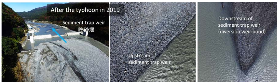
Fig. 6 Sedimentation at the upstream and downstream of sediment trap weir of Miwa
