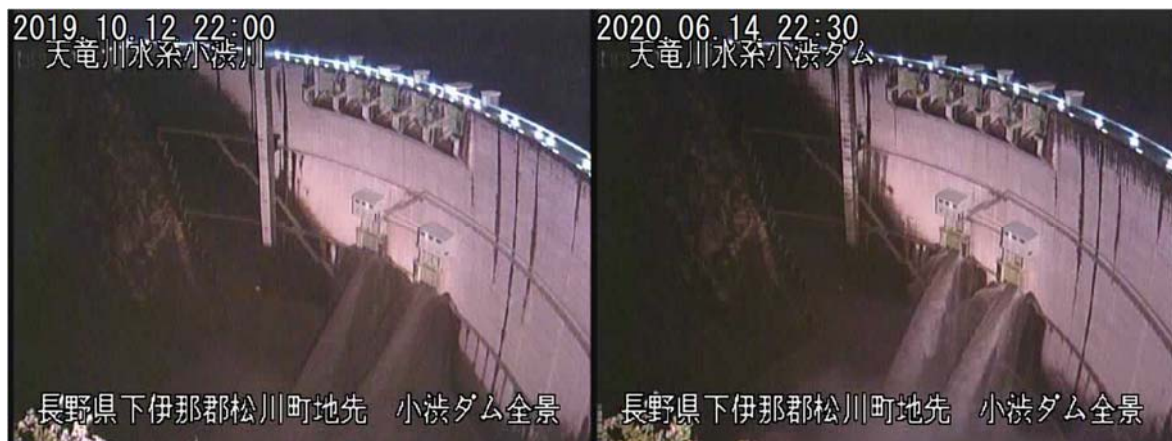
Fig. 8 Flow release from conduit gates of Koshibu during the typhoon (left) and different flood (right).
