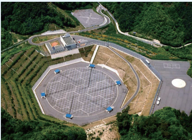
MU radar antenna the first large-scale MST radar with a two-dimensional active phased array antenna system Completion: 1984 Size: 103 m in diameter Award: selected as IEEE Milestone
