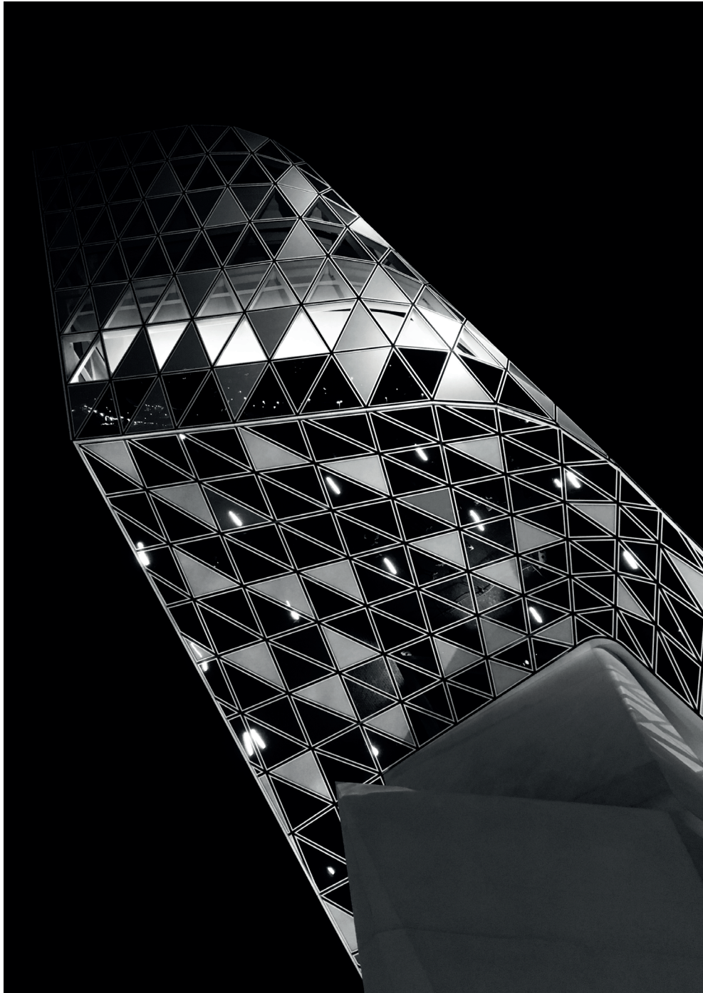
Port House (Antwerp, Belgium)
