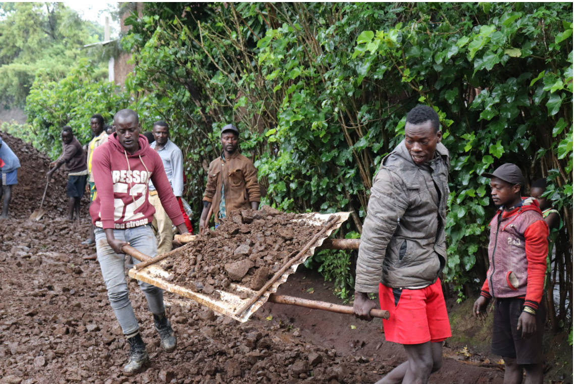
4. Villagers Scattering the Gravel in Pairs. Since the Path Was Narrow, They Scattered Manually. Jinka. December 2019
