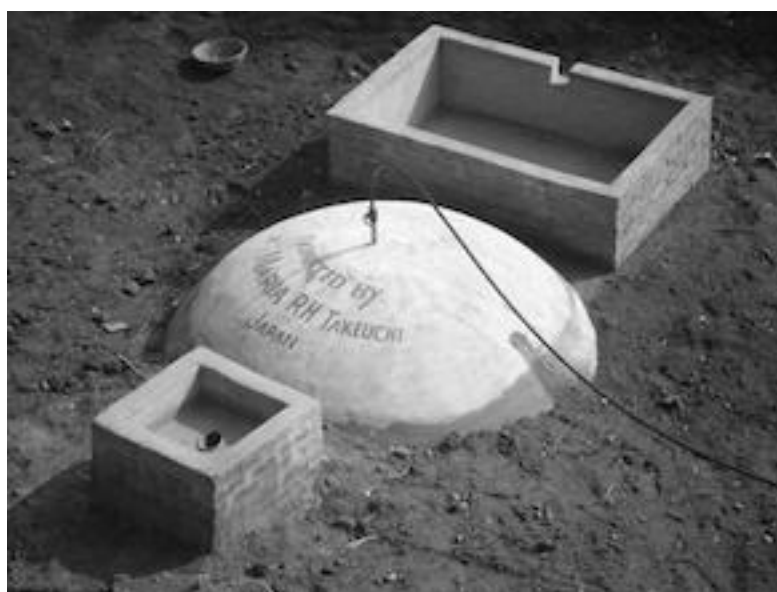
Figure A.1. Small biogas plant in a village
