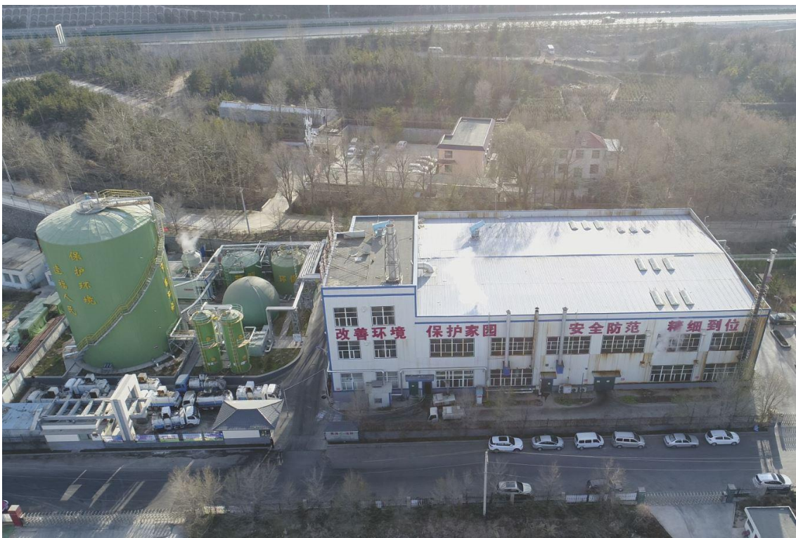
Figure A.4. Working biogas plant in China
