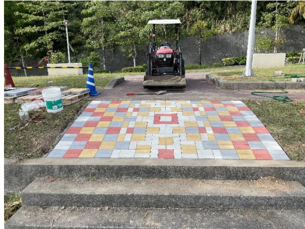
Figure 5 Construction site after laying interlocking concrete blocks
