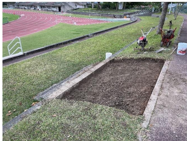
Figure 3 Construction site after dug
