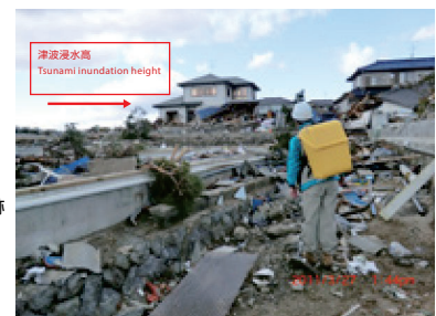
宮城県七ヶ浜町での津波痕跡と調査の様子 Tsunami trace and survey in Shichi-ga-hama coast in Miyagi Prefecture
