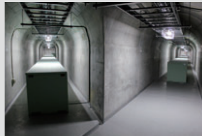
2016年に竣工した桜島の高免観測坑道 Underground tunnel to detect precursory ground deformation to eruptions, newly constructed in 2016
