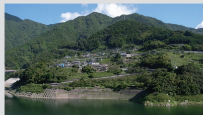
四国山地における典型的な地すべり(地震計による観測斜面) Typical landslide in the Shikoku Mountain (with earthquake observation by means of seismometers)
