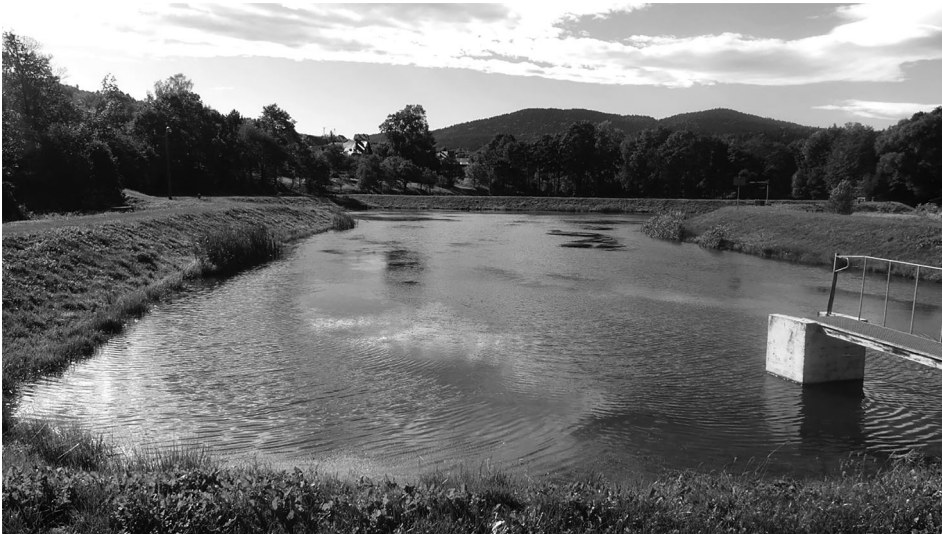
Figure 3. The reservoir in Wiśniowa (Source: Authors).
