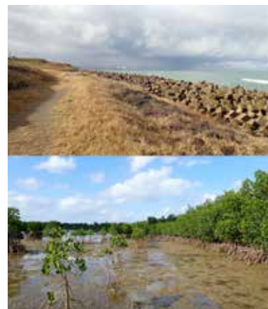
Figure 1 Examples of gray and green infrastructure in coastal environments: top – breakwaters along the Ogata coast (Niigata, Japan); bottom – mangrove forests in Iriomote Island (Okinawa, Japan)
