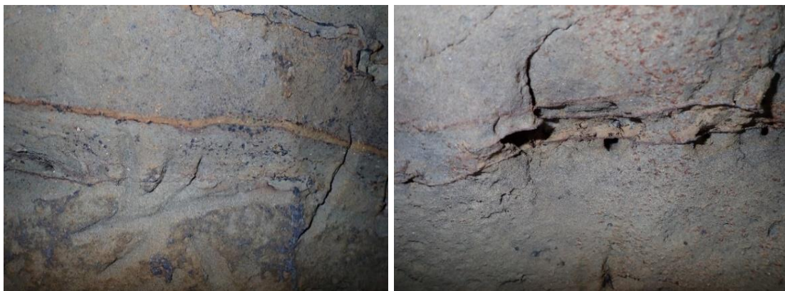
Figure 6.6. Hydrated iron oxide precipitation on wall of the Yokoana tomb No.16
