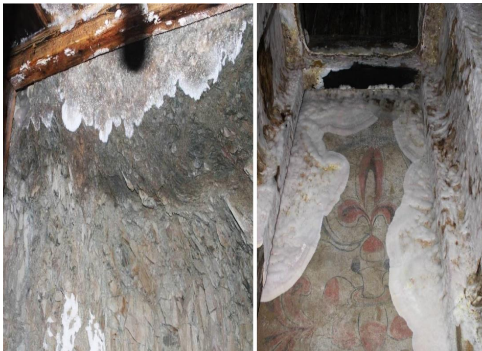
Figure 4.2. Fungus developing on surface of the mural painting in the airshafts and burial chamber
