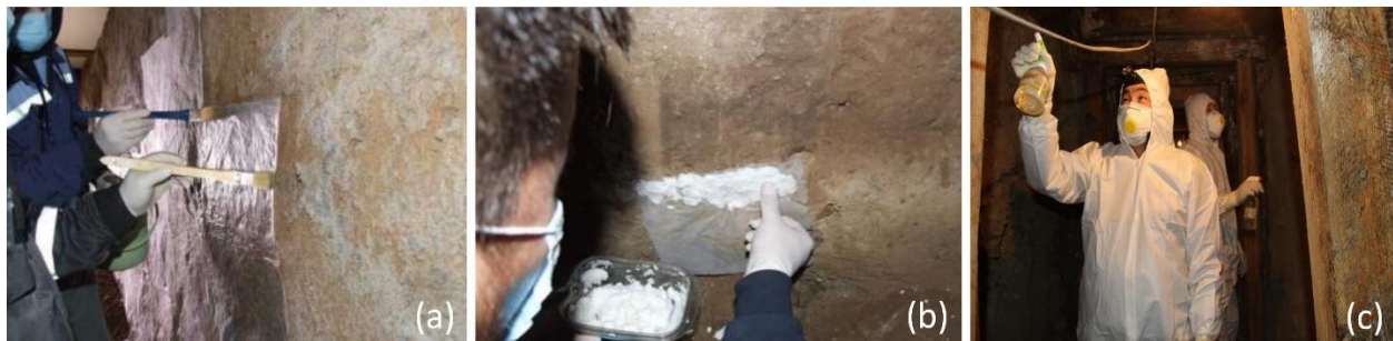
Figure 1.4. Preservation-Conservation workshop (UNESCO). a) Re-positioning of paint layer detachment, b) Desalination test, c) Removal of microorganisms from wooden propping
