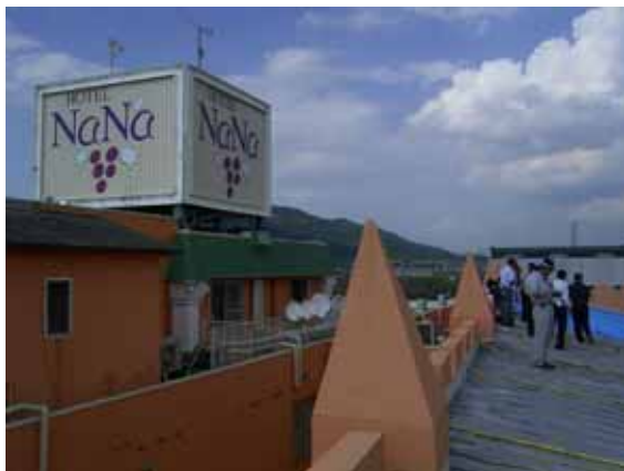
Photo 5 Damaged roof (Right) and control building (left).
