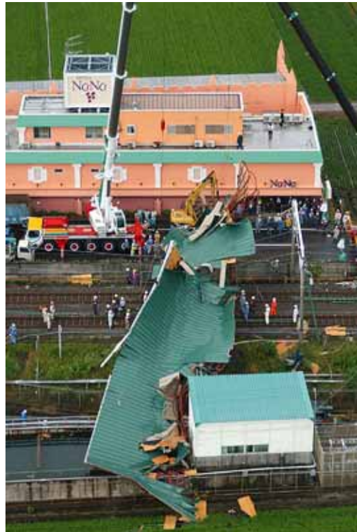
Photo 1 Blown Roof of a hotel onto the JR track.
