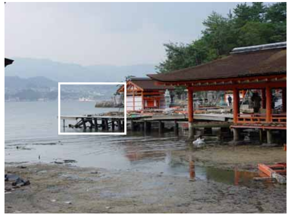
b. Site of collapsed Sagakubou
