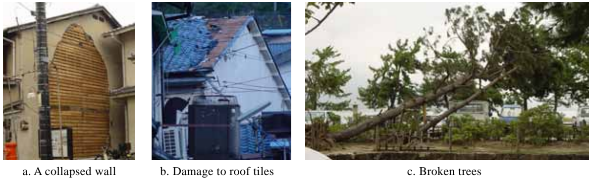
Photo 3 Various finds of damage recorded around Itsukushima Shrine in Miyajima Island
