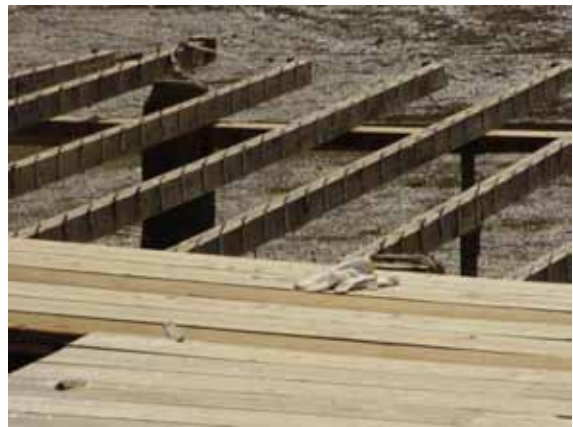
g. Joists and posts of Hirabutai
