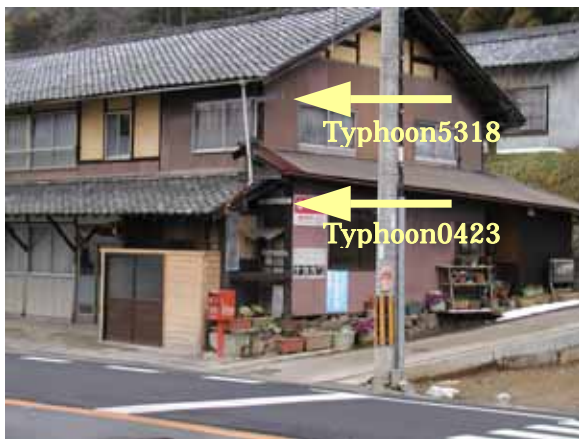
Photo. 3 Flood marks on a house near Okumo bridge
