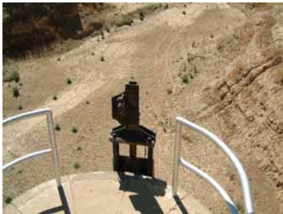
Photo 4 Empty reservoir of Ikrimah dam
