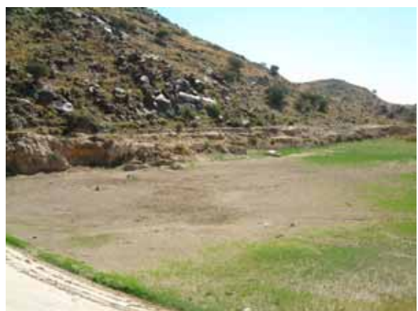
Photo 6 Empty reservoir of the rockfill dam
