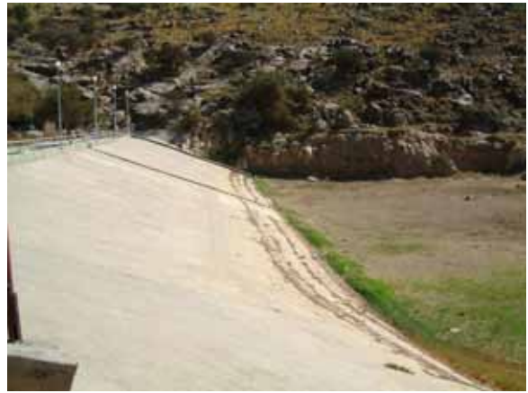
Photo 5 A facing type of rockfill dam
