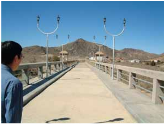
Photo 3 Crest road of Ikrimah dam
