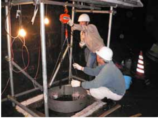
Photo 2 Setting work of the strainmeter
