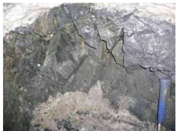
Photo 1 Hard rock into the hole excavated
