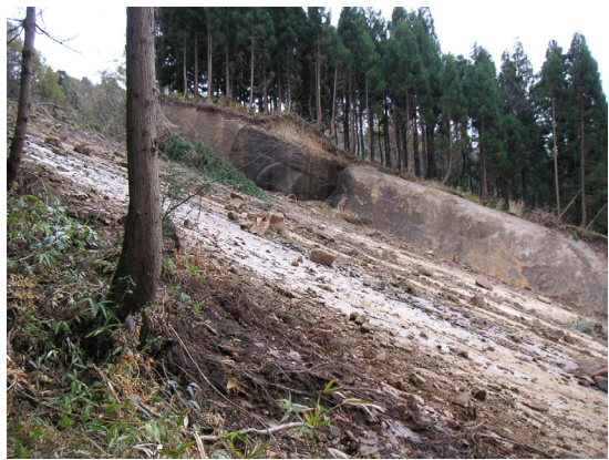
Photo 2 Slope collapses at Yokowatari area. (enlarged photo)
