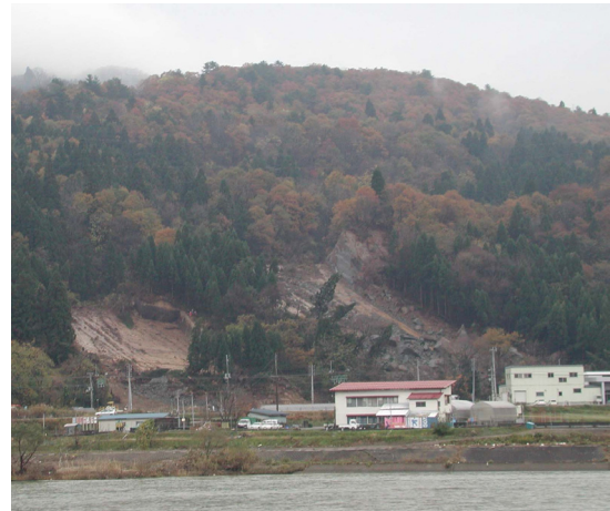
Photo 1 Slope collapses at Yokowatari area
