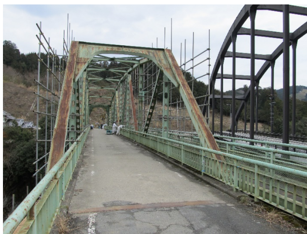
Figure 21 Overview of the bridge
